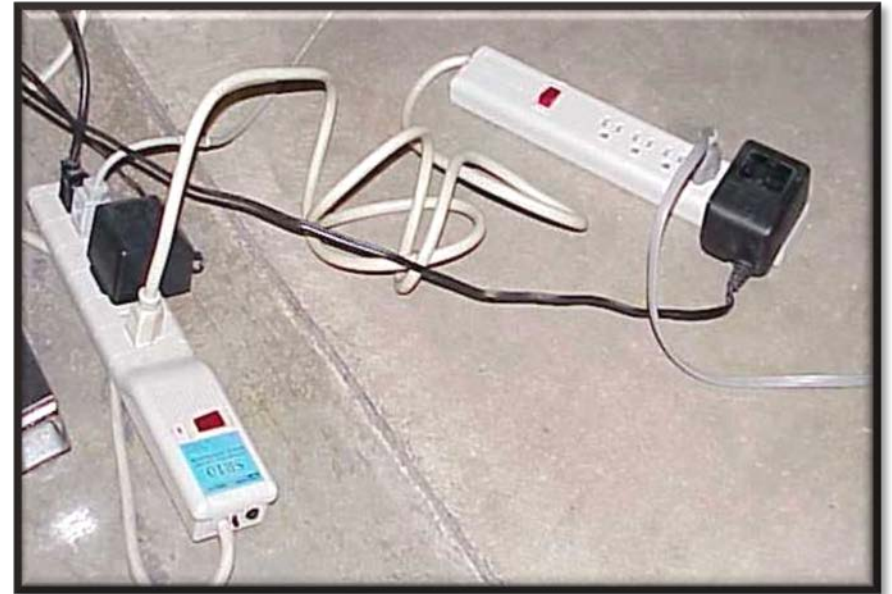
Do not use piggy-backed multi-plug strips
